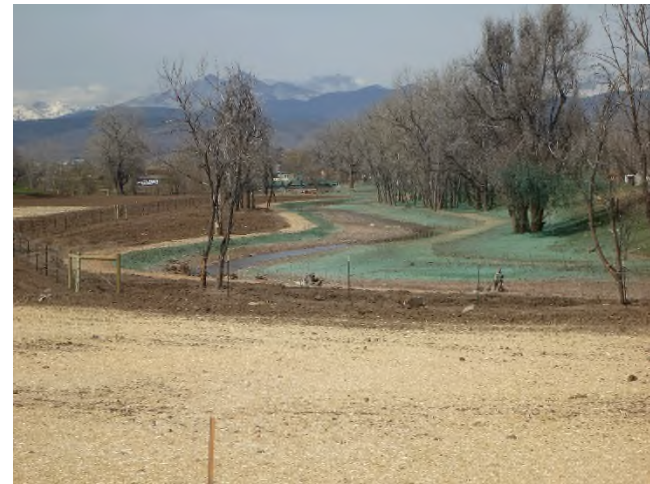
Figure 2 – Looking upstream from the downstream end of the project reach. Hydro-mulch has been applied to the zone 1 seeding area as well as the left overbank (photo right). The completed fence on the Jackson property is shown as well.
