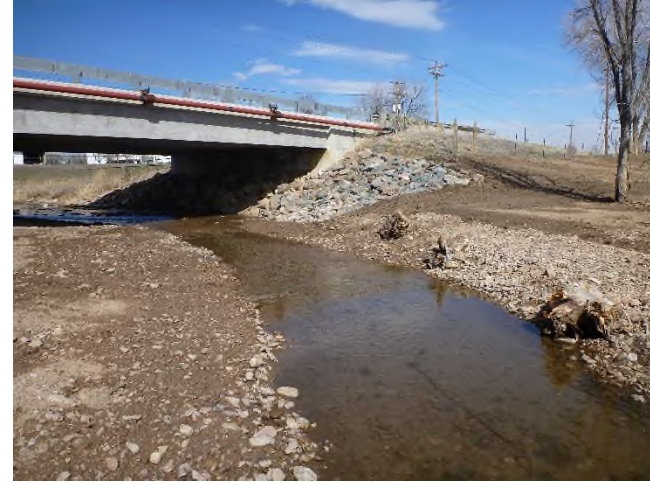
Figure 1 – Looking downstream near Sta 0+50 at the design reach tying into the existing undisturbed channel at the County Road 4 bridge.
