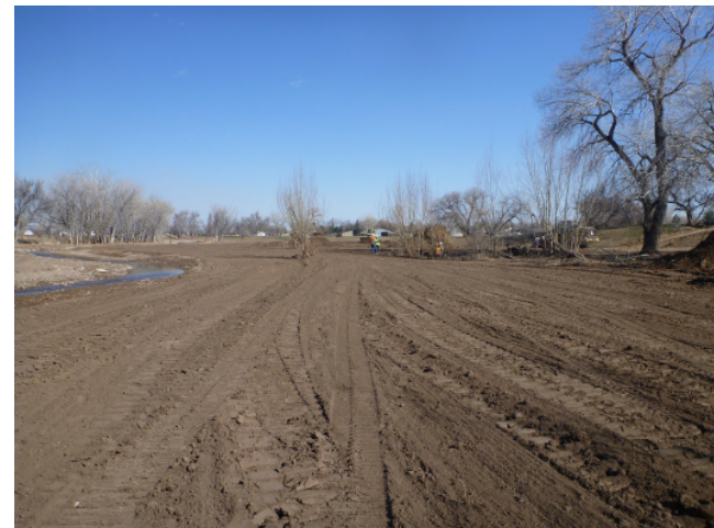
Figure 2 – Looking downstream near Station 14+00 at the newly graded right overbank.
