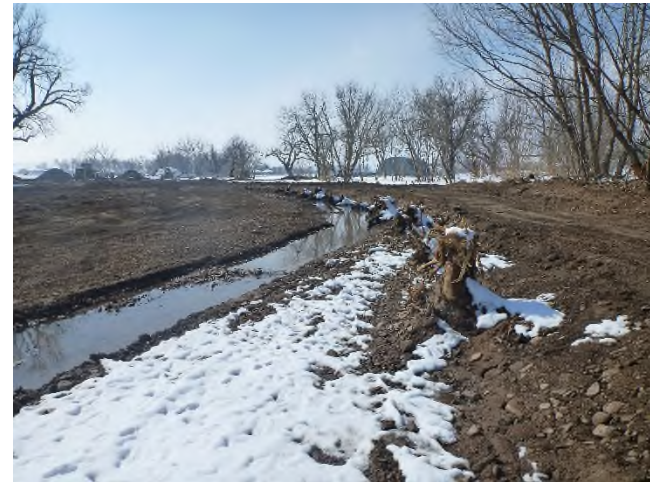
Figure 2 – Looking upstream from Sta 17+00 at the recently completed rootwad revetment on the left bank (photo right).
